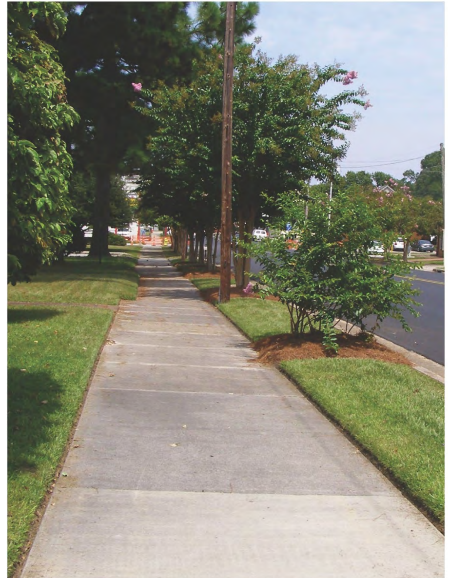
Buffered sidewalk facility, Whiteville, NC (Image Source: HCP).
